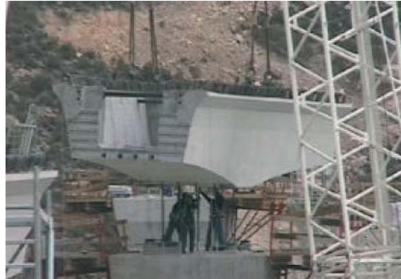
Fig. 17: Piece in cantilever over the pier
