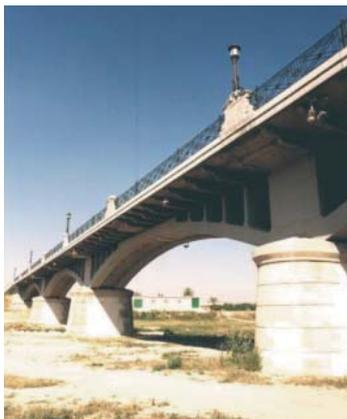
Fig. 23: Precast concrete arch bridge
