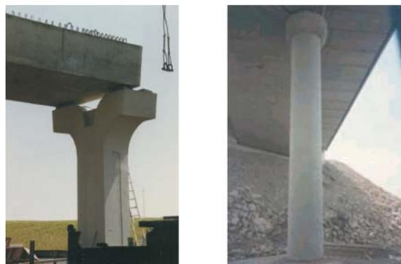
Fig. 12: Precast bridges with mono-beams
