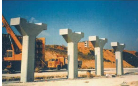
Fig. 45 to 47: Piers of independent columns with simple and double capital
