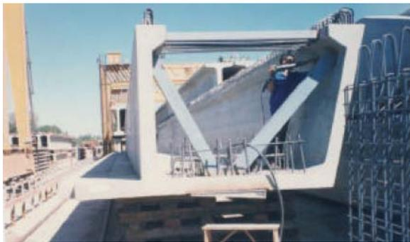
Fig. 28 & 29: U-beam for railway bridge with longitudinal joint to form a triclular box
