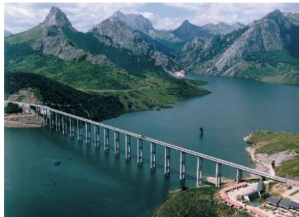
Fig 50: Precast bridge with piers 65 m tall
