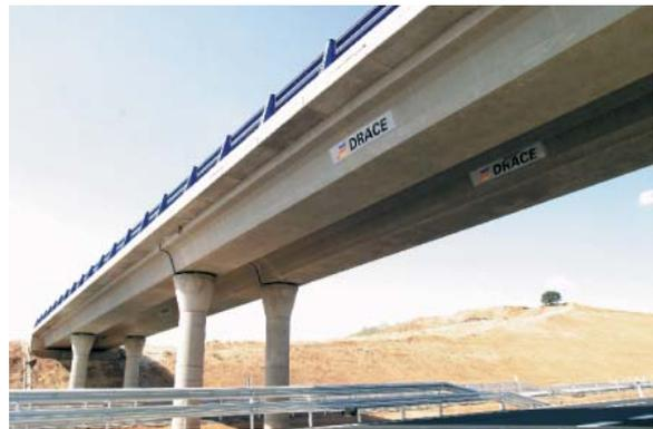
Fig. 11: Precast bridge with U beams deck
