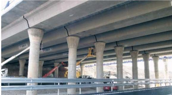
Fig. 26: Bridge with decks of U-beams
