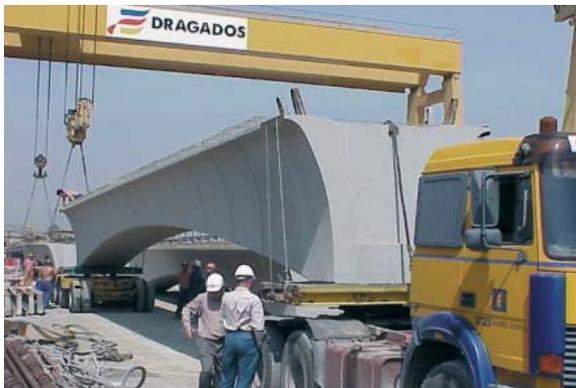
Fig. 14: Transport of variable height U beam
