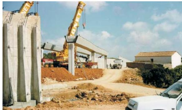
Fig. 44: Abutments of cantilever counterfort elements
