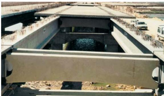
Fig. 32 & 33: Precast deck slabs of full thickness
