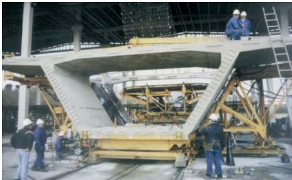
Fig. 35: Segment of full transversal section at the precast plant
