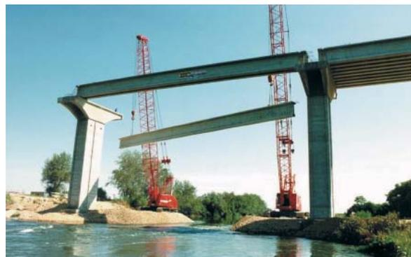
Fig. 24: Bridge with decks of I-beams
