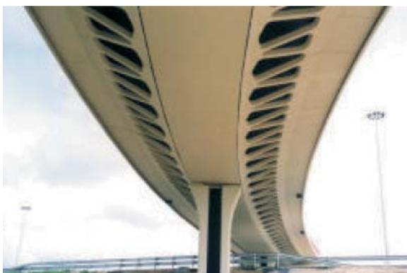
Fig. 16: Diagonals of complex shape
