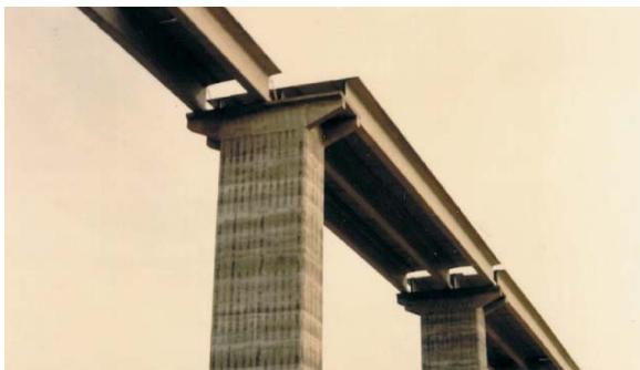
Fig 48: Precast crossheads on site cast piers
