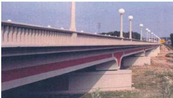
Fig. 22: Precast bridge with special shape
