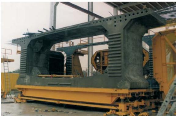
Fig. 36: Segment of partial transversal section
