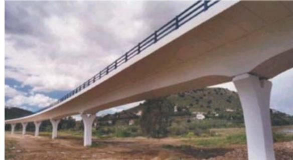
Fig. 27: Bridge with decks of mono-beams of curved layout and variable height
