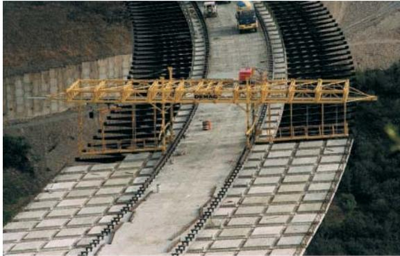
Fig. 34: Precast deck slabs of full thickness on steel structure (box girder & diagonals)
